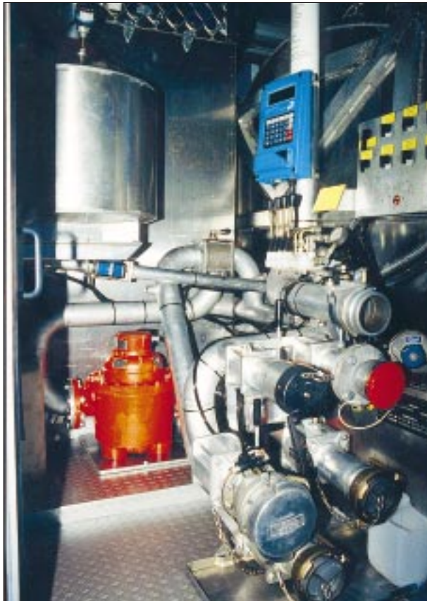
Fig. 2 Control room and pipe fittings
